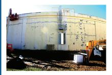
The old ladder from the floor to roof hatch was removed and new ladders at each of the two manholes will be installed after the walls are coated with a flexible internal spray-on liner (CIM) which will stop the leaks through the original tank wall. The exterior painting will likely begin in the spring 2013 due to winter weather conditions and the dome roof fall protection system will be installed after the exterior painting.
