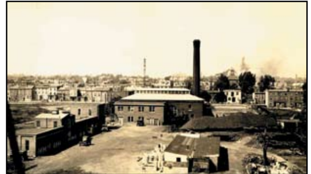
Original Pumping Station in City of Chester, early 1900s
